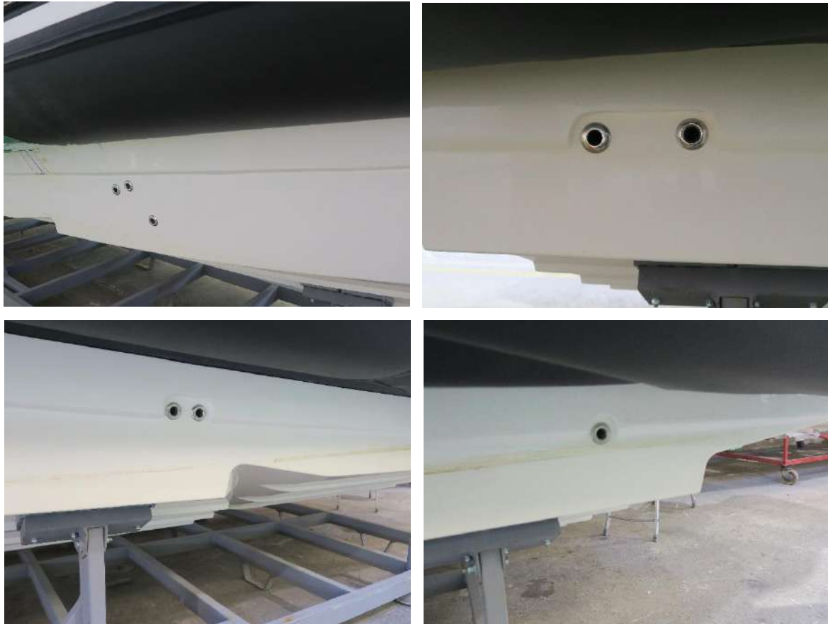
Detailed view of the through-hull fittings
