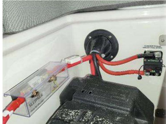
Windlass circuit breaker and fuse
